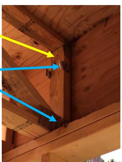
A plumber destroyed this truss by removing structural members and making numerous penetrations to the Top & Bottom Chord.
