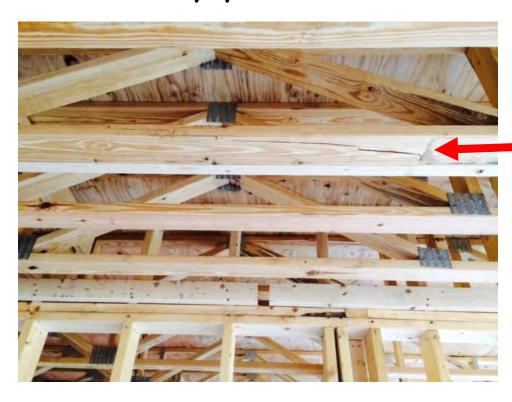
The Bottom chord of the Truss is cracked.
